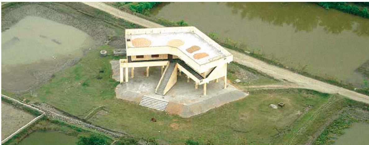
Photo: A multi-purpose cyclone shelter
